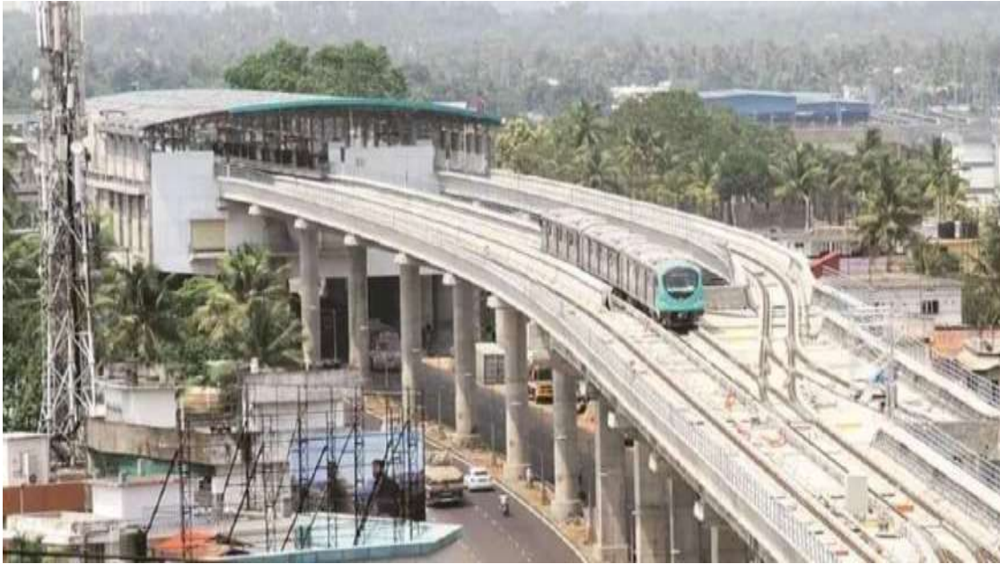
Figure 1: Kochi Metro Rail Project
