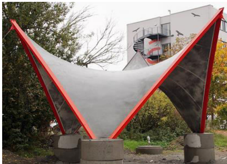
Figure.2. Shows the flexible Bendable Concrete structure.
