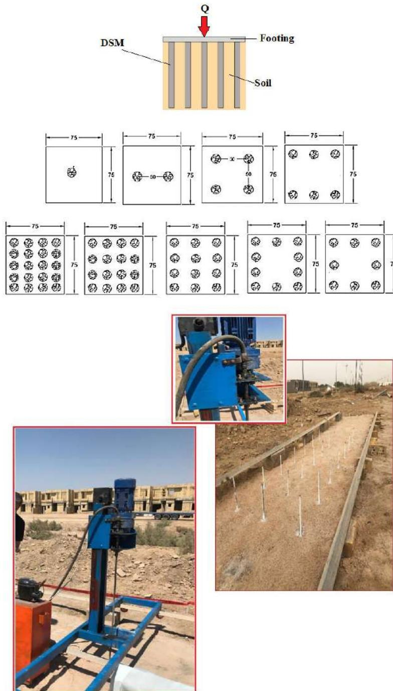
**Figure 2:** Configuration of the field tests and site work
