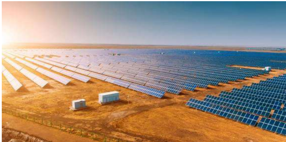
Figure 1: Large-Scale Photovoltaic Solar Farm in an Region
