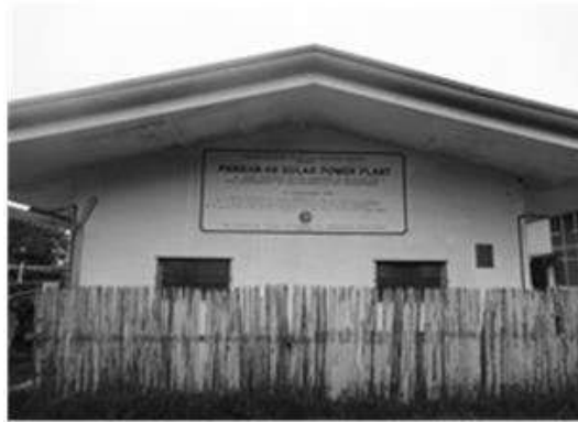
Figure 1. Pangan-an Solar Power Plant
