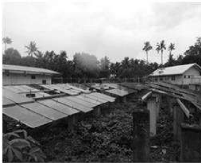
Figure 4. Vegetation Growing Near Solar Panels
