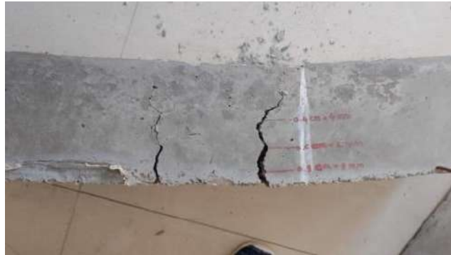
Fig 10: Crack Pattern for 100% RCA beam
