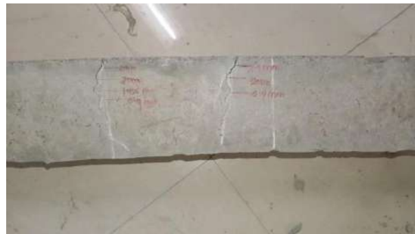
Fig 11: Crack Pattern for 50% RCA beam
