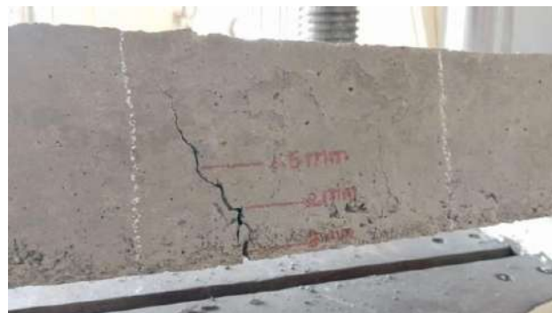
Fig 12: Crack Pattern for 0% RCA beam
