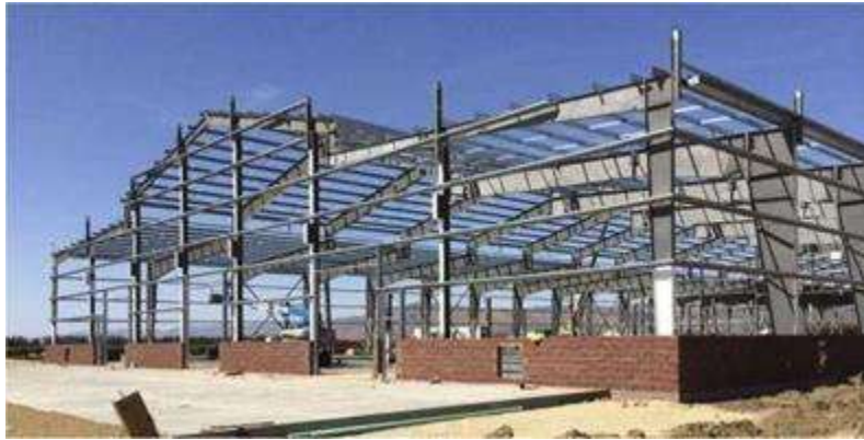
Figure 1: Pre-engineered steel building
