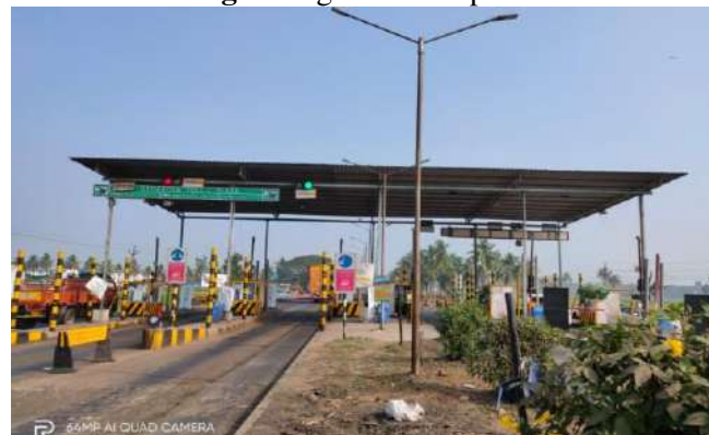
Fig. 6 Ethakotha Toll plaza
