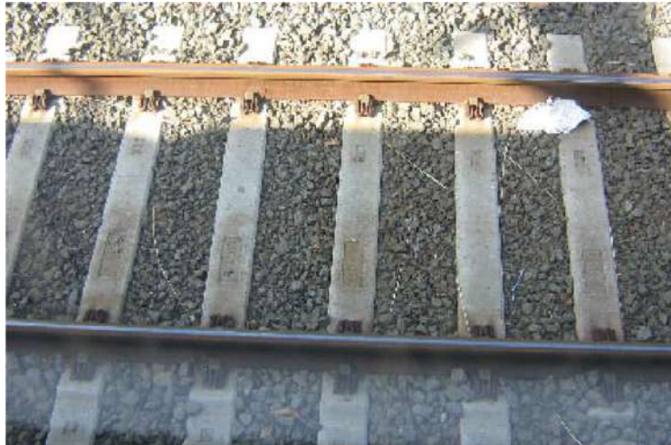
Fig.2 Partial Replacement sleepers
