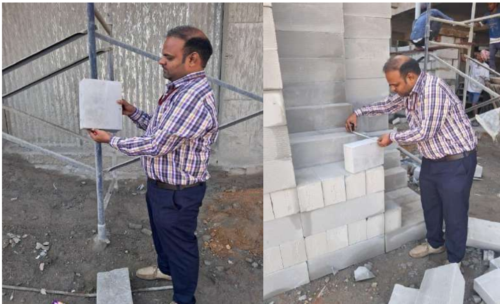
Figure 3: Dimesional check on site for AAC Blocks
