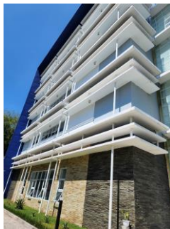
FIGURE 2 SHADING DEVICES OF A BUILDING
