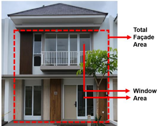
FIGURE 1 WINDOW TO WALL RATIO (WWR)
